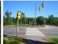
Crossing Pullen Road
