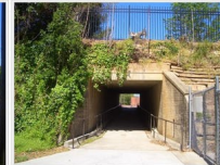
Tunnel under Morrill Drive
