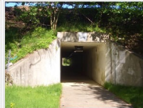
Tunnel under McDowell Street
